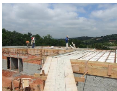
concreting the roof
